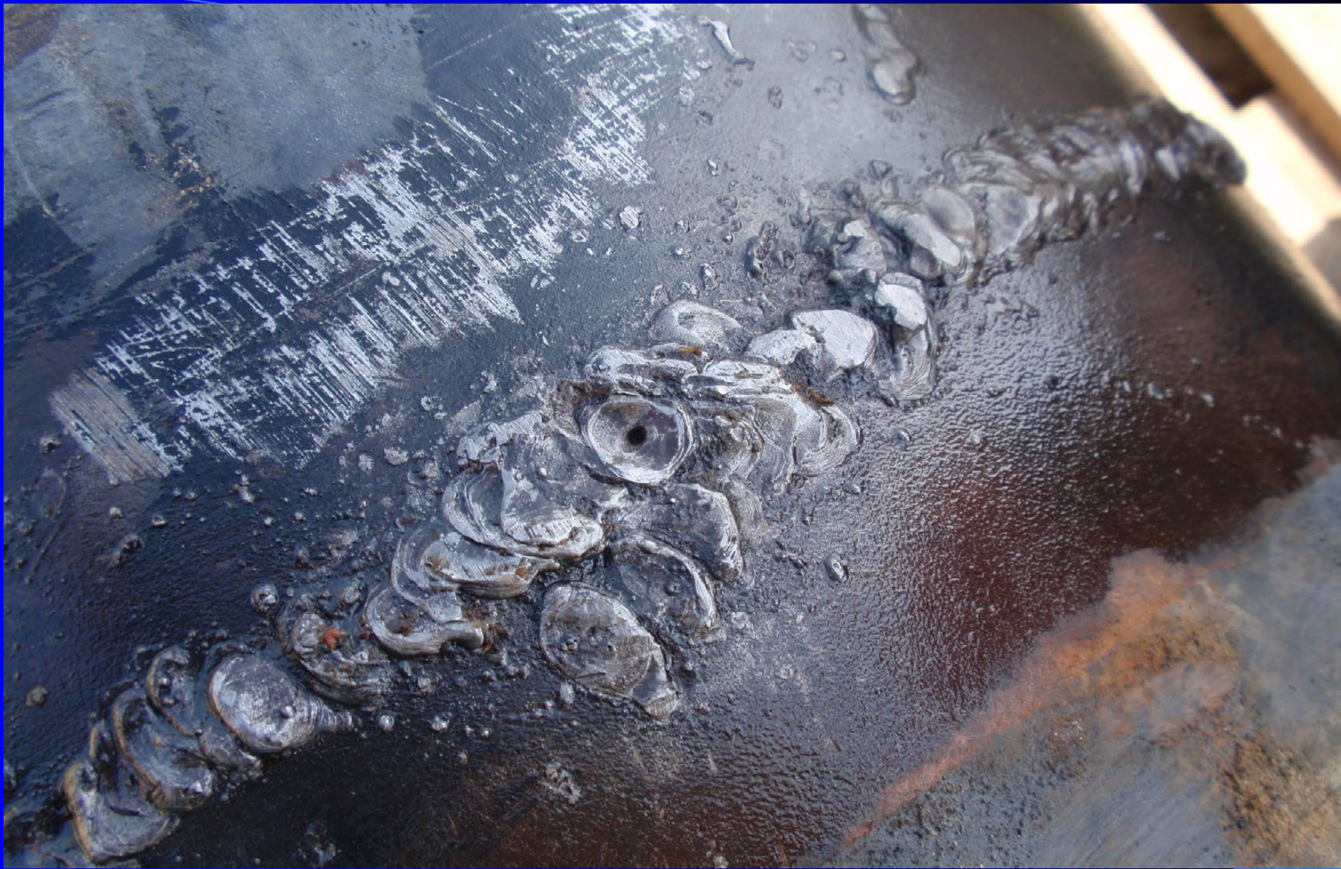
Assembly weld with defect
