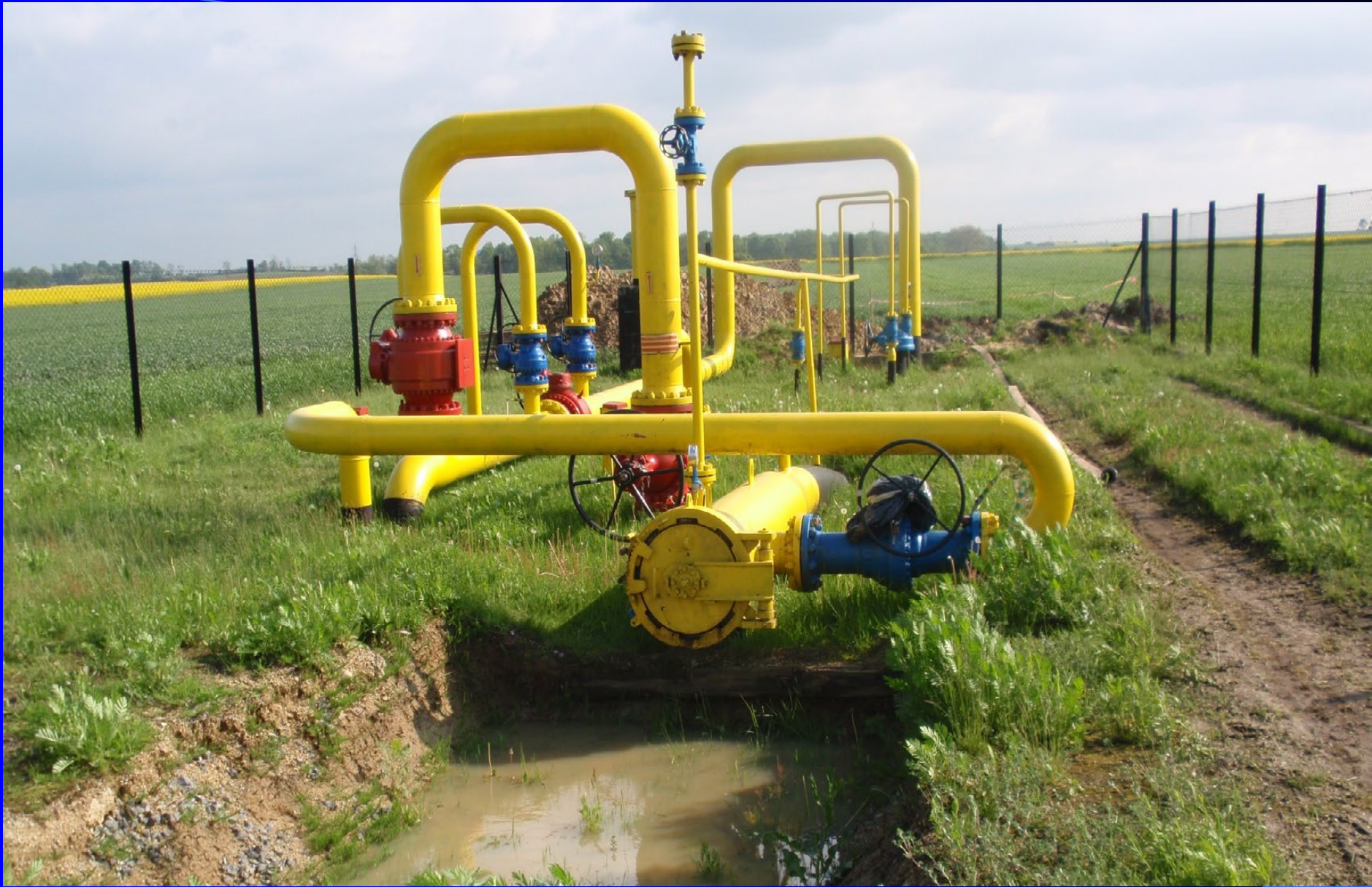
Launching trap in the beginning of pipeline
