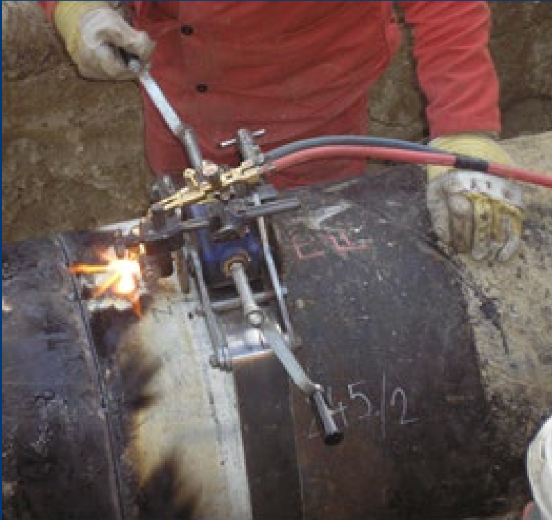
Flame cutting at permanently explosion safe conditions
