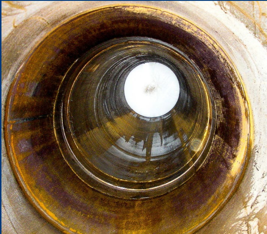
Internal pipeline surface after cleaning
