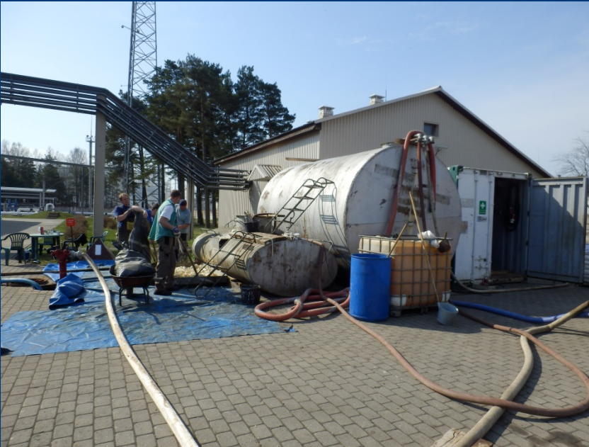
Preparation of PETROSOL water solution on jobsite
