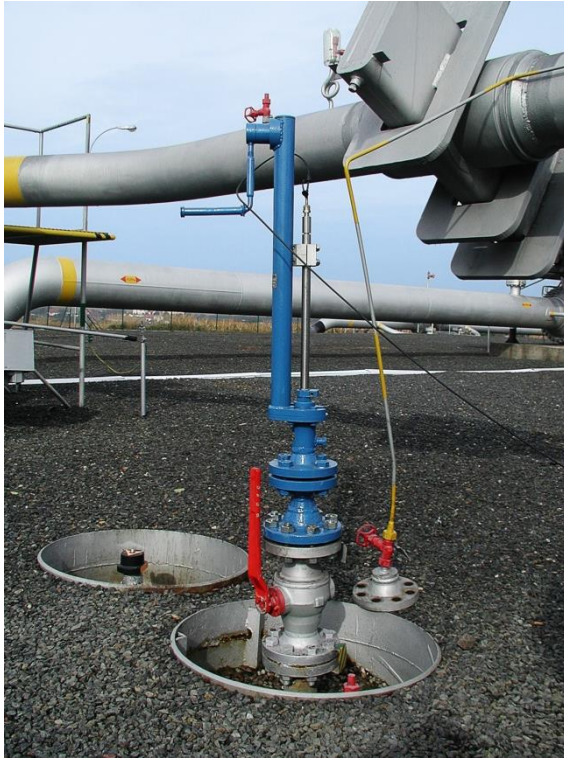
The probe taking gas samples from the pipeline
