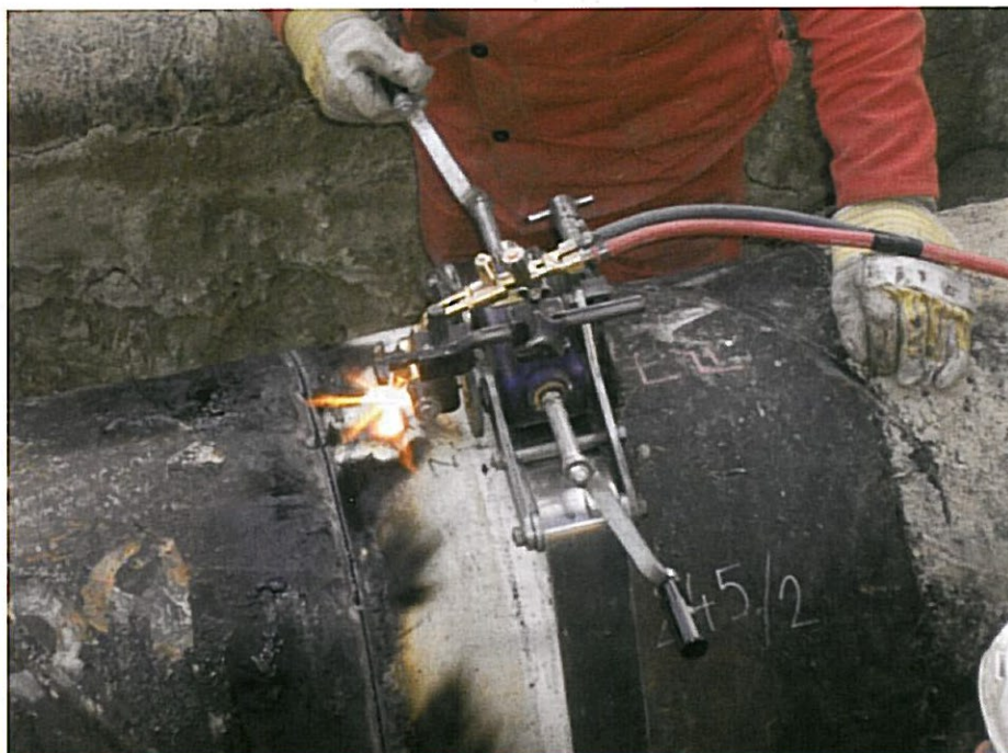
Pipe cut-out using oxyacetylene flame.
