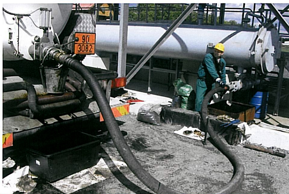
Displacement of oil from the 28 inch diameter pipeline into road tankers.
