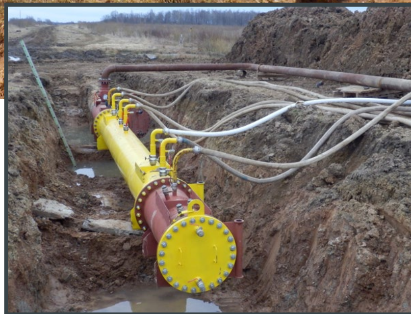
Figure 5: Launching trap with the water supply pipeline and hoses
