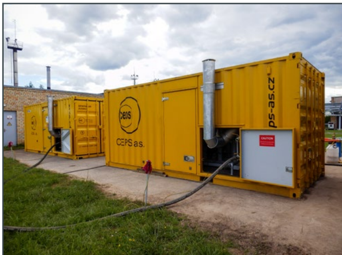
Figure 3: CEPS mobile nitrogen generators
