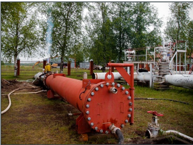
Figure 4 and 5: Temporary traps for chemical cleaning
