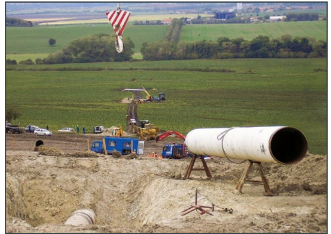
Figure 10: Spread of some jobsites
