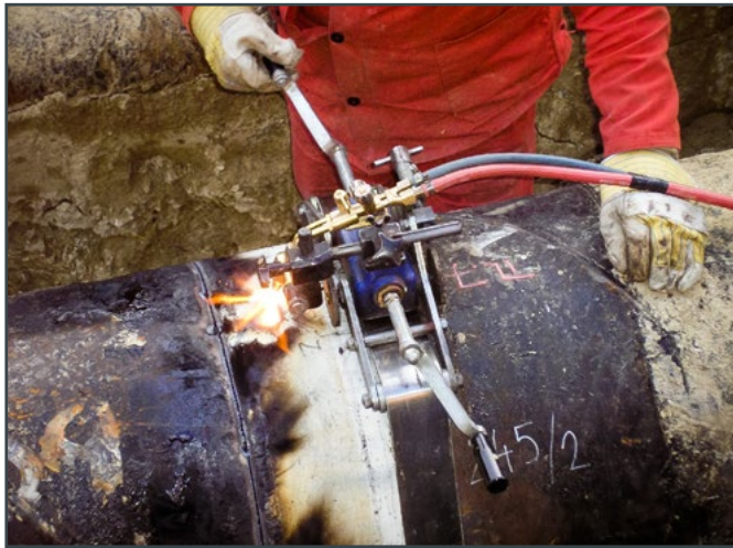
Figure 8: Flame cutting at permanently explosion safe conditions
