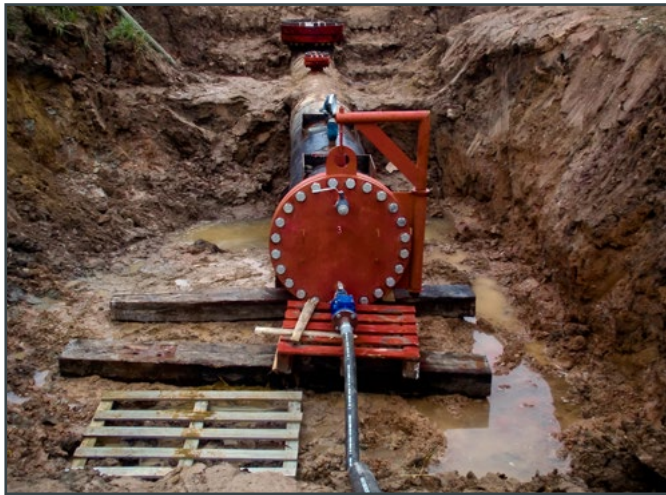
Figure 2: CEPS temporary launcher trap
