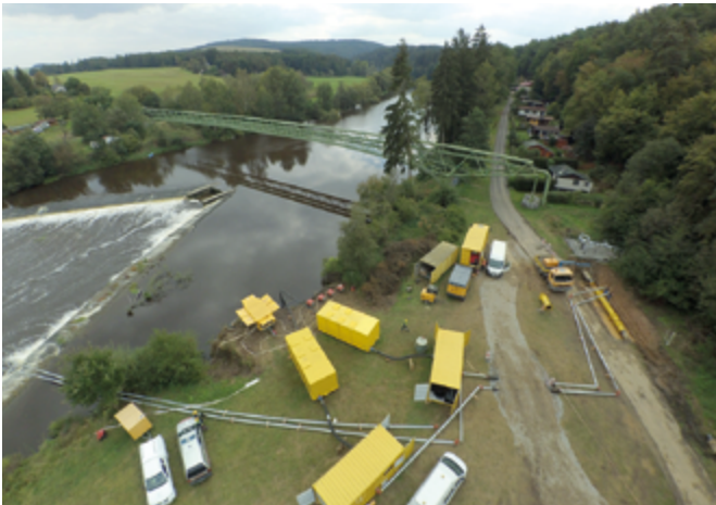
Obr. 11. Staveniště u Borečnice Fig. 11 The site near Borečnice
