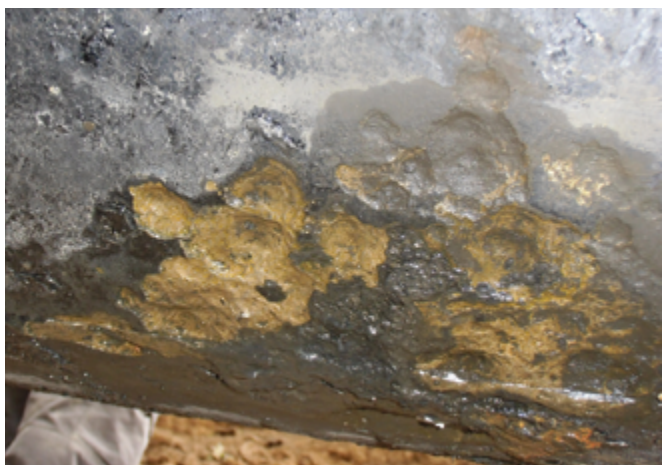
Obr. 1. Koroze potrubí DN 600 Fig. 1 Corrosion on the DN 600 pipeline
